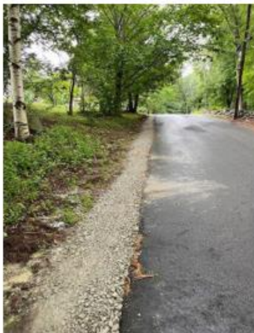
Moulton Ridge Road July 2021- Road Shoulder Repair
