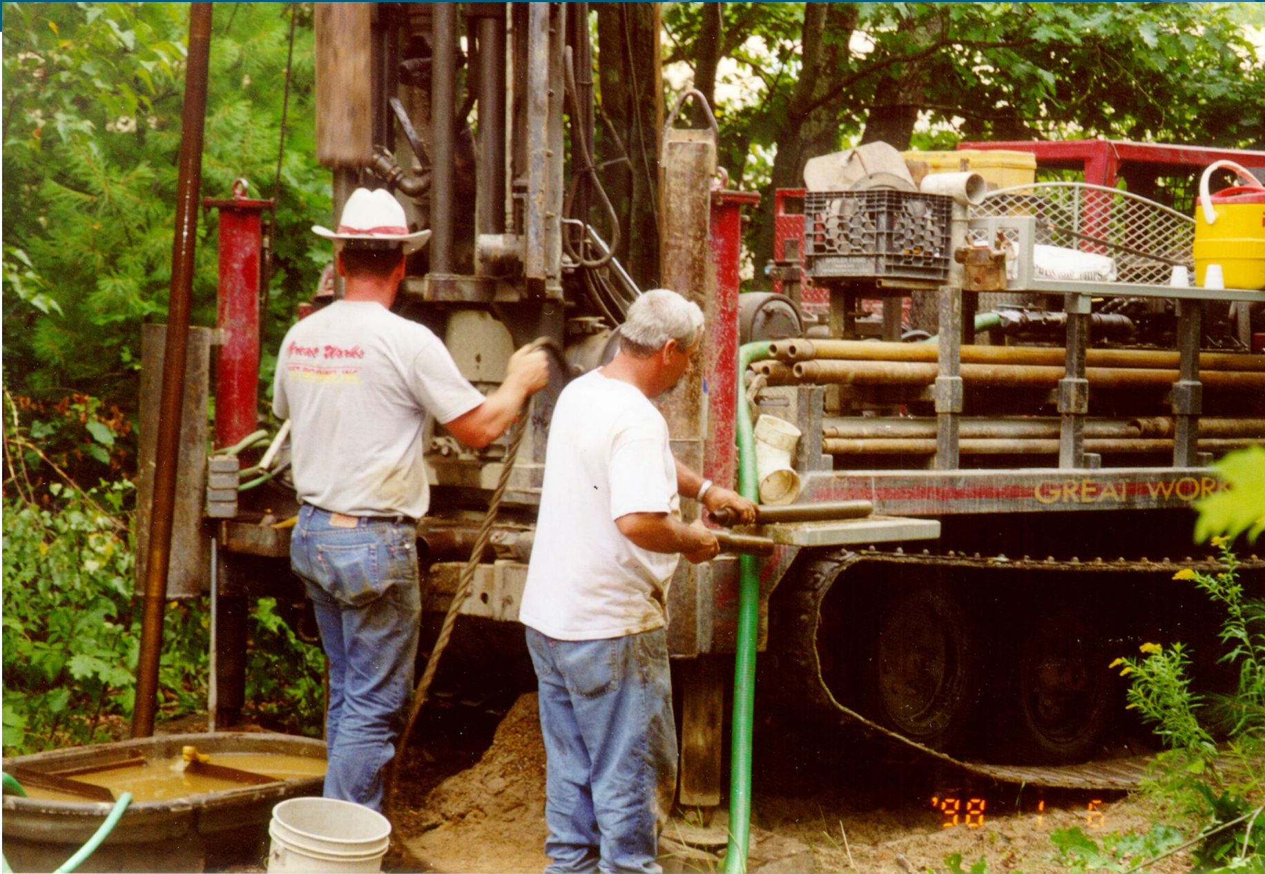
Emery & Garrett Groundwater Investigations, A Division of GZA
