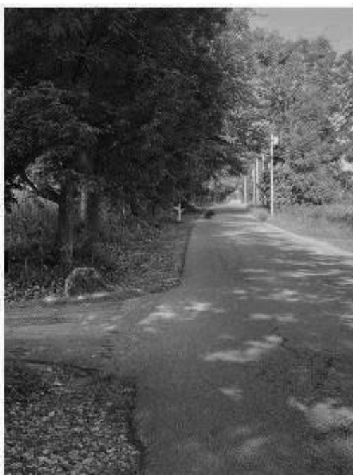
Stumpfield Road, August 2022- Ditch line Repair
